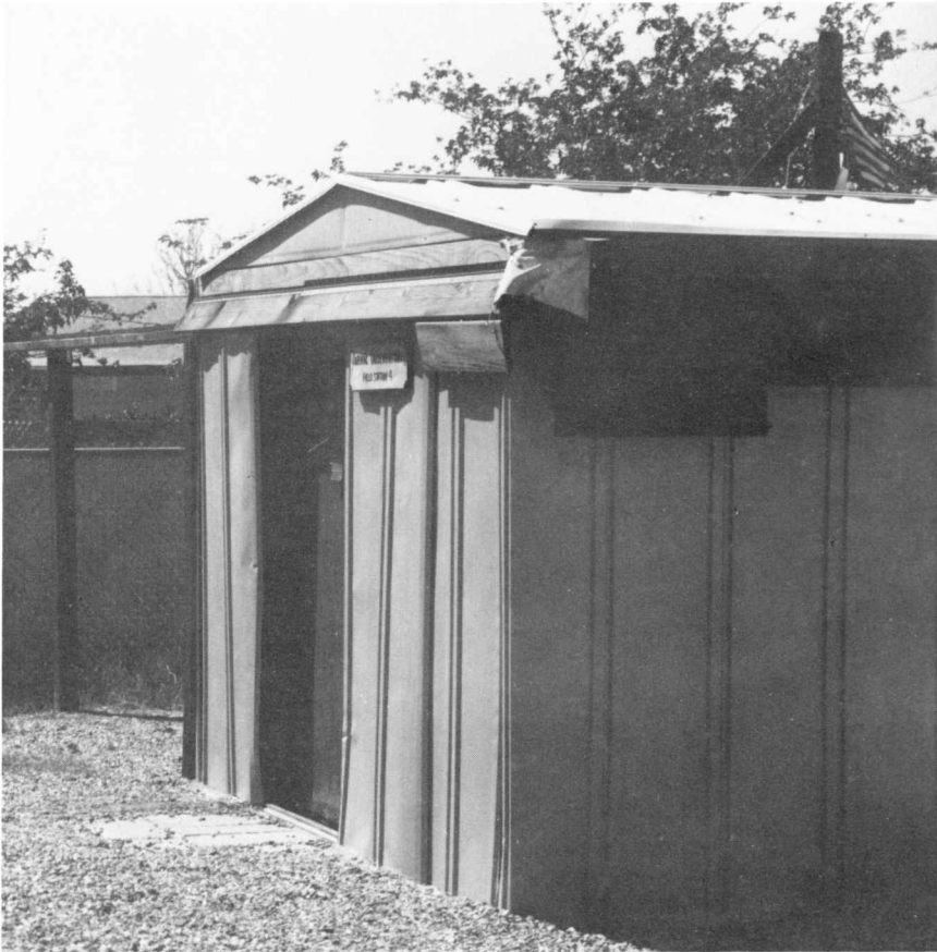
FIG. 2. Station “4” – an observatory building for the 0.4-m reflector. The telescope housed here is now my main observing instrument.
