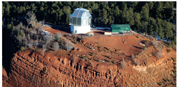
Figure 3 — Aerial view of the DCT dome and support buildings.
