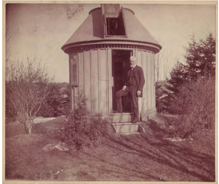
Figure 2 — John Goldie outside his observatory in Galt. His equatorially mounted refractor is visible through the open door and dome. The structure is typical of small 19th-century observatories, although the woodwork and finish appear to be quite superior. The design, known as the “Romsey Observatory,” is the Victorian equivalent of the SkyShed POD. It was developed by the Rev’d Edward Lyon Berthon (1813-1899), and was meant to be a solid, adaptable, low-cost alternative to other structures. The design would probably work as well today as in the days of Queen Victoria (Berthon 1864). The Romsey Observatory would have been a familiar sight on the 19th- and early 20th-century Canadian astronomical landscape; have any survived?
