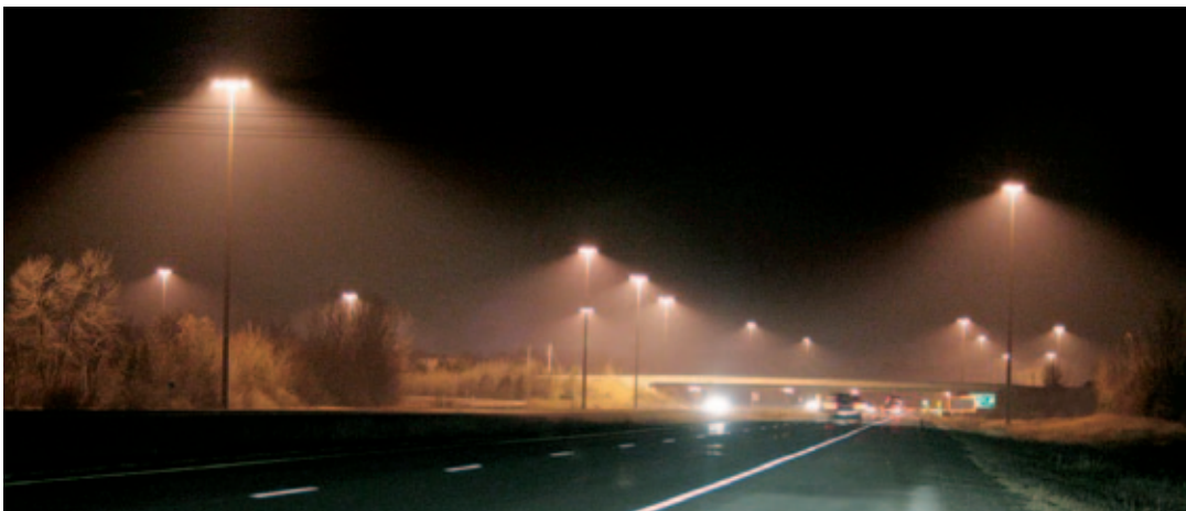
Roadway lighting highlights an area where heightened attention is needed, such as in this interchange with Hwy 416 and Hunt Club Road in western Ottawa. These full-cut-off luminaires improve visibility while limiting the impact on the surrounding forest and open fields. (Nov. 2011, R. Dick)
