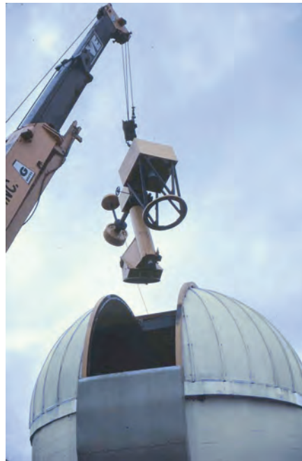
Figure 3 — Loading the dome: the new telescope frame is lowered into place in the Tabor Mountain observatory.
