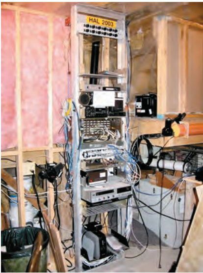
Figure 7 — “HAL 2003.” The rack contains the operational heart of Radio Jove, the meteor detection system, and video and network distribution for the building and all the piers.
