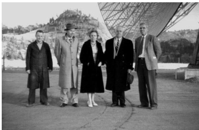
Dr. C.S. Beals, the Dominion Astronomer, visited the staff during the early days of construction. L to R — John Galt, Ed. Argyle, Kaye Adams, Dr. Beals and the author. Missing is Roy Hamilton — who took the picture.
