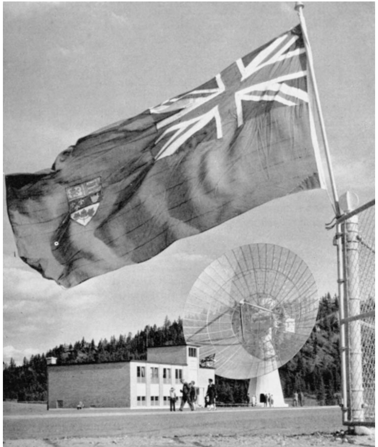
Dominion Radio Astrophysical Observatory, White Lake, Penticton, B.C., showing the 84-foot radio telescope and the office building on opening day, June 20, 1960. (Photo by Penticton Herald .)
